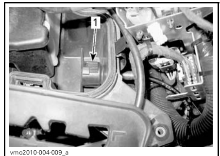
1. ACS compressor air filter
