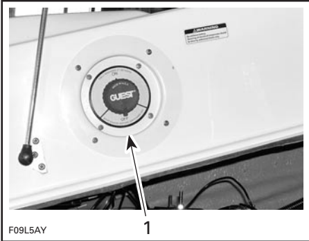
TYPICAL — MAIN BATTERY CUT-OFF SWITCH 1. Battery cut-off switch in OFF position
