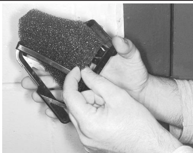
REMOVAL OF FILTER FROM ITS GRILL
