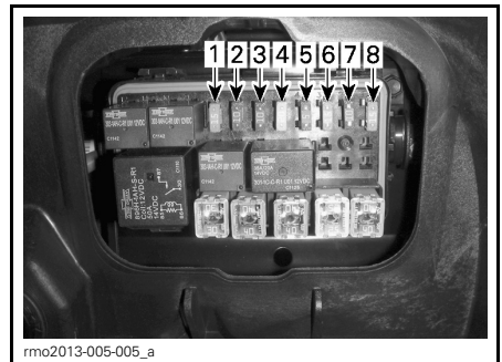
FUSES - LEFT FUSE BOX
