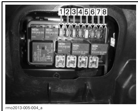
FUSES - RIGHT FUSE BOX
