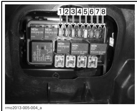
FUSES - RIGHT FUSE BOX
