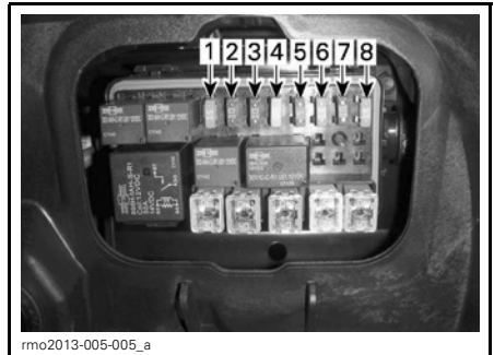
FUSES - LEFT FUSE BOX
