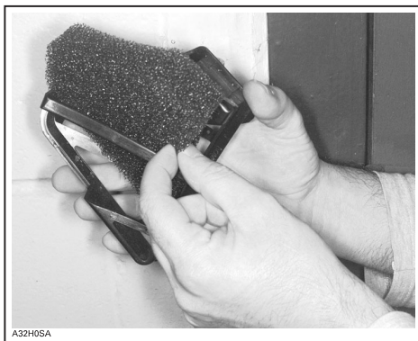
Removal of filter from its grill
