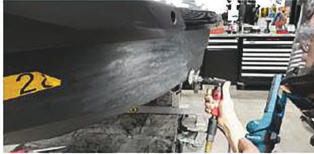
Transition area in work.
