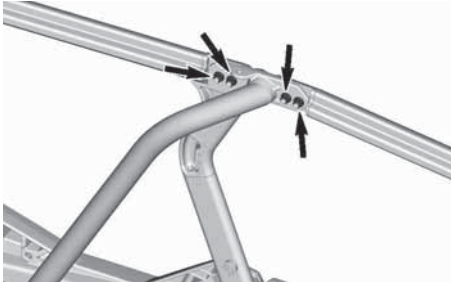
TOP OF CENTRAL PILLAR
