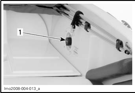
1. Main battery cut-off switch
