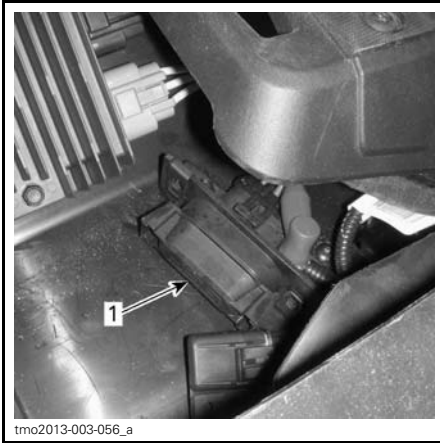
1. Auxiliary fuse box
