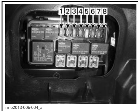
FUSES - RIGHT FUSE BOX
