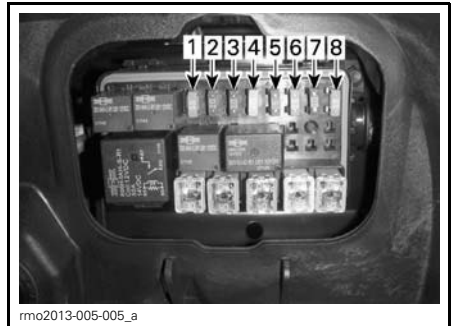
FUSES - LEFT FUSE BOX
