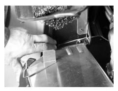
Lift cover front side up and bend it to out from unit to get it removed.
