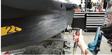
Transition area in work.
